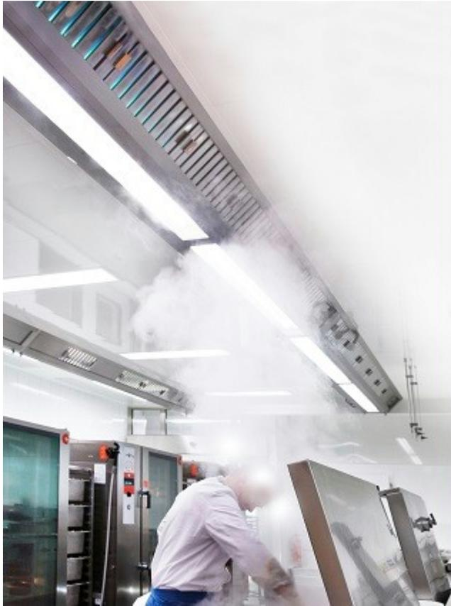
Everybody knows it: The smell of roasting and frying in the kitchen. The odour not only gets into your nose but the fat contained in the fumes also leaves traces in the kitchen. UV technology solves this problem lastingly. Grease and smells in the exhaust duct are photolysed and cleaning is made easier.
